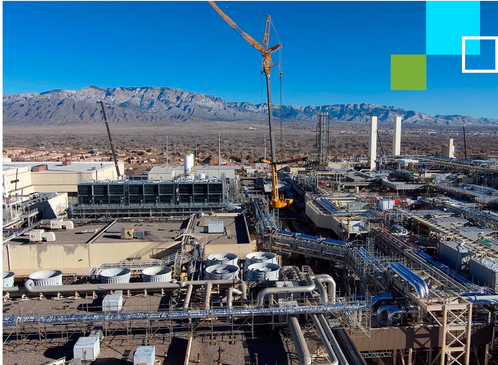
Construction underway at Intel's site in Rio Rancho, New Mexico.
